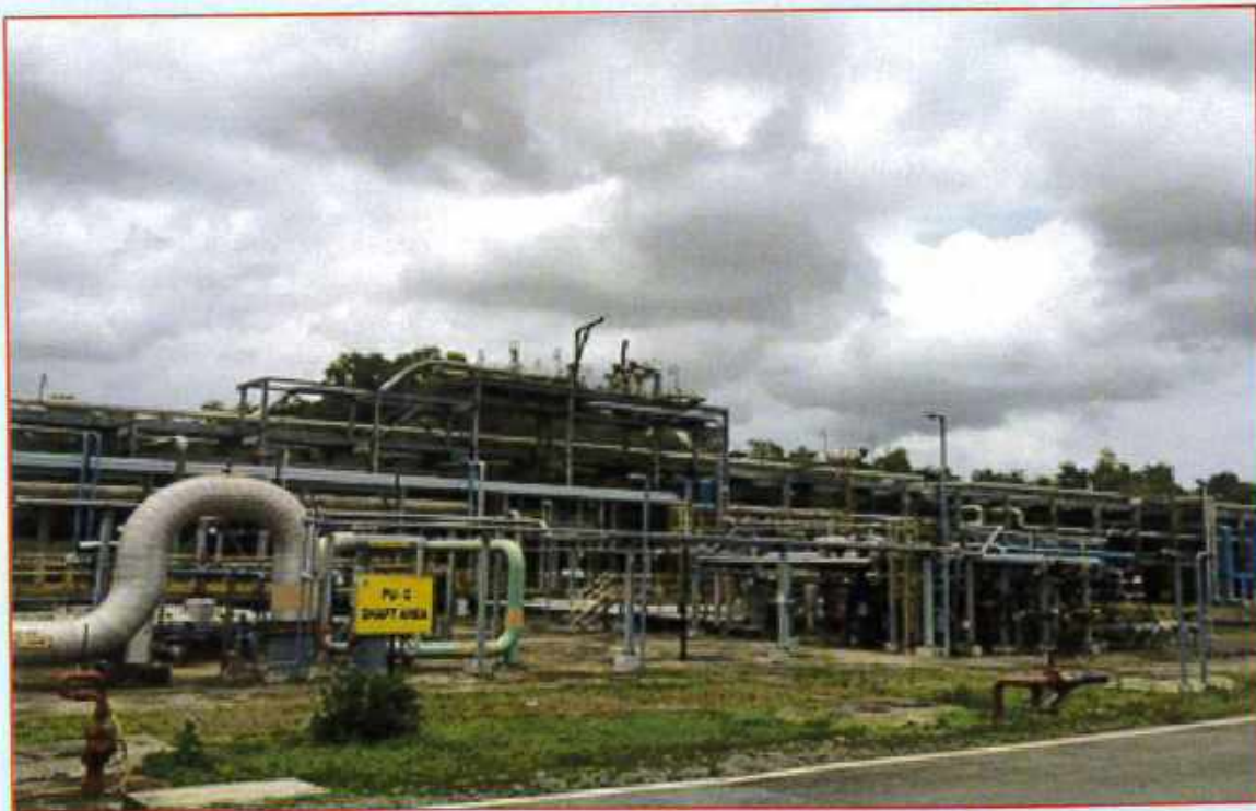
View of above ground facilities at cavern area
